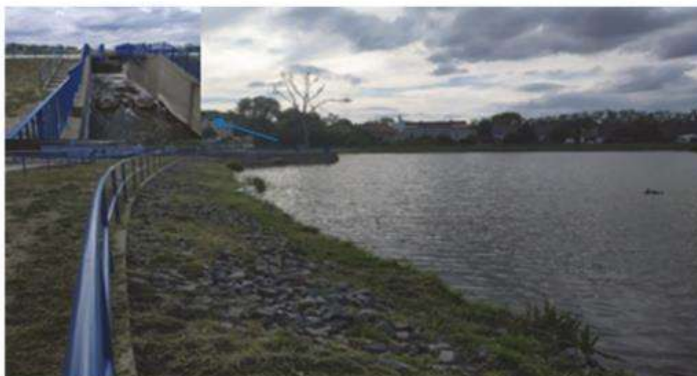
Fig. 2. The embankment dam with the spillway-overflow structure (steady level damming) in the Przebędowo reservoir
