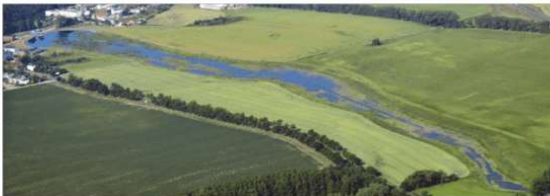
Fig. 3. A view of the Przebędowo reservoir (Sojka et al. 2017)
