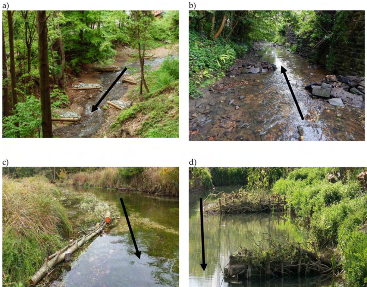
Fig. 1. Examples of different deflector design solutions, a) deflector development with logs and stone erratics of the Roztoka Mała mountain stream bed (PCW, 2018), b) stone deflector system on the Königsseer Ache mountain river, Austria (rivercale.org, 2021), c) D-shaped wicker deflector on the lowland river Skerne, UK (wildtrout.org, 2021), d) fascine silage deflector – the lowland river Welland UK (bristolavonrivertrust.org, 2021)
